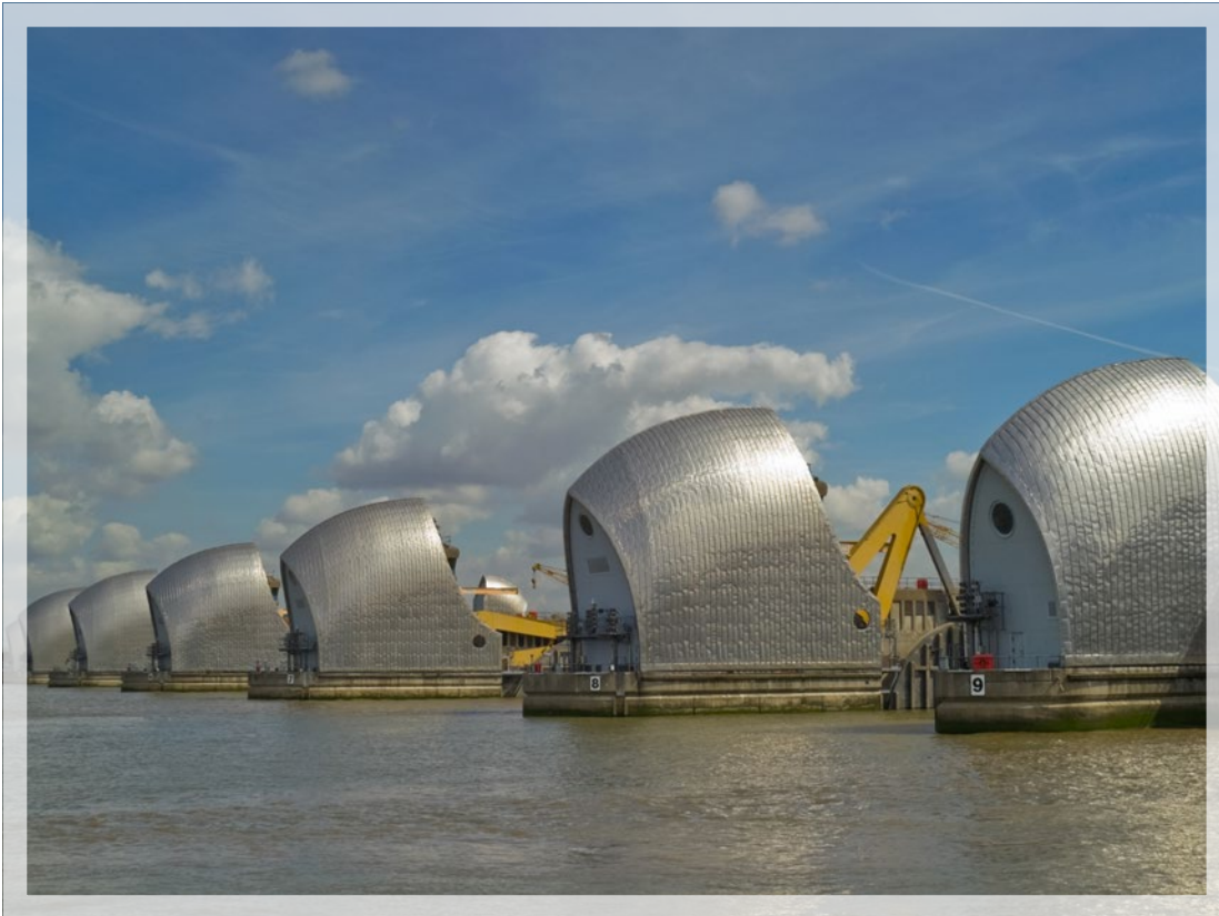
Fig. 22.1. The Thames Barrier is a movable storm surge barrier constructed in 1982 to protect London (Photo: Rui Saraiva/Shutterstock).
