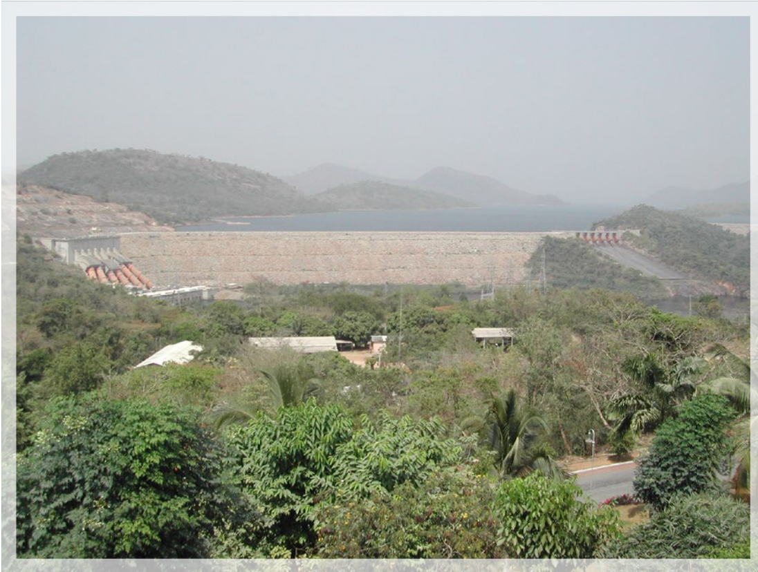
Fig. 14.1. The Akosombo dam in Ghana has dramatically reduced the sediment supply to the coast from the Volta River.
