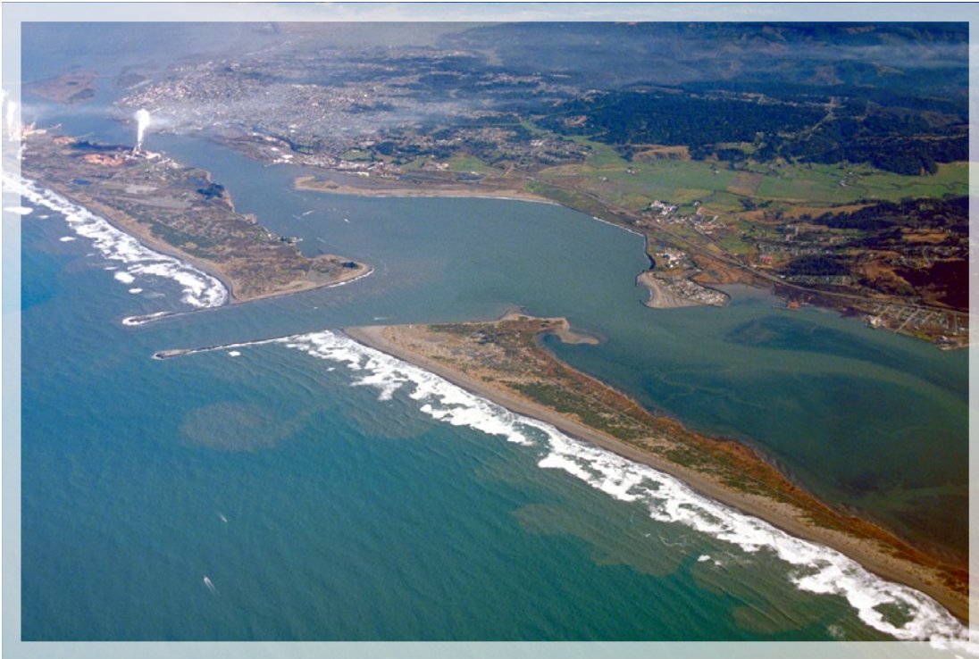
Fig. 17.1. Jetty structures in California (Photo: U.S. Army Corps of Engineers Digital Visual Library 2007, CC BY-SA 3.0).
